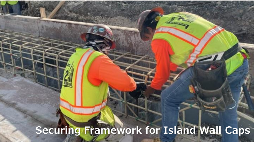
July 2023 Installing Island Walls
